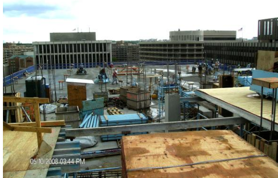
View of 13 th floor west pour (area 2) from 14th floor east (area 1) framing, 2 days after 13 th floor east pour (area 1).
