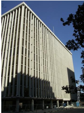
Exterior façade to be removed
