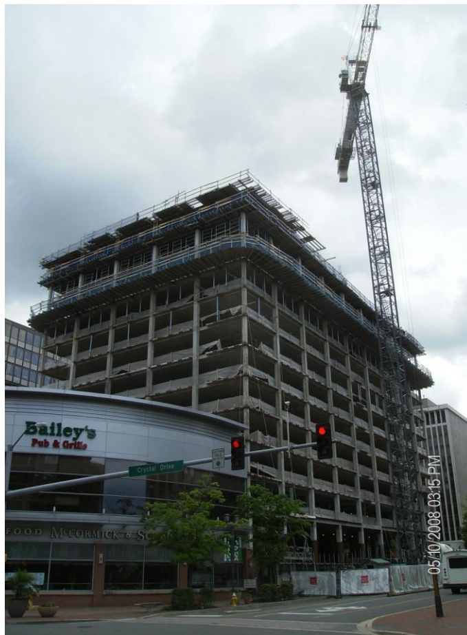
Superstructure and Glazing Phase beginning
